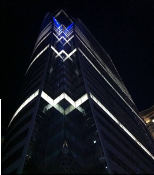
Sathom Square – Gold LEED standard accreditation. DJCoalition has experience in achieving accreditation under Nabers, Greenstar and LEED.
